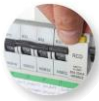
Consumer unit (fuse box or trip switch)-
